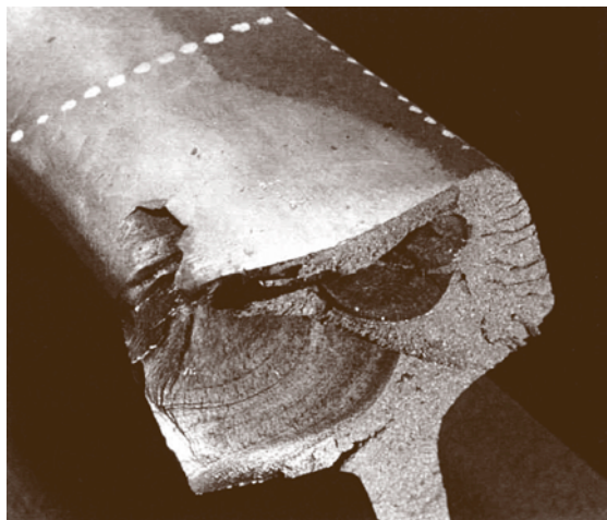
Fig. 16.27 Broken rail caused by head checks
