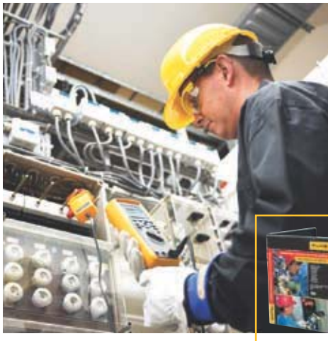
Use protective equipment such as safety glasses and insulated gloves
