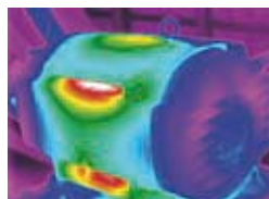
Abnormal/uneven heating on motor
