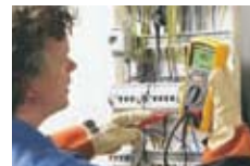
Insulation test at a distribution panel
