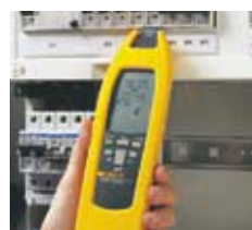
Location of fuses/breakers and assignment to circuits
