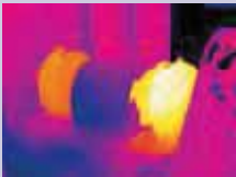
Overheating bearing cap
