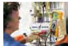
Insulation test at a distribution panel
