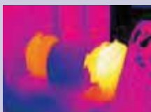
Overheating bearing cap
