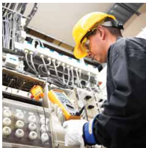
Use protective equipment such as safety glasses and insulated gloves
