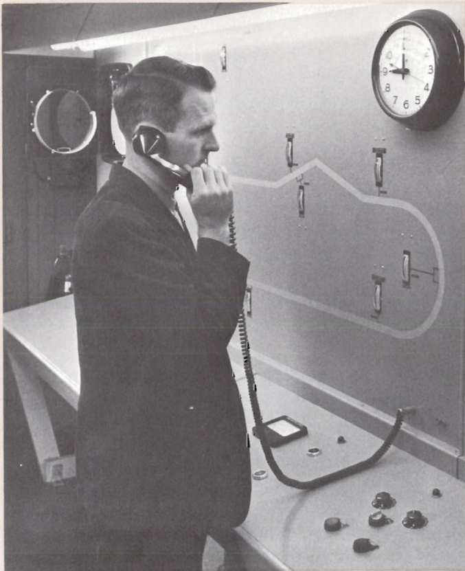
Operator stands at control panel where diagram shows layout of pipeline system and data check points.
