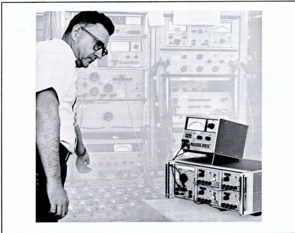
FIGURE 8. Calibrating Production Line Standard with an E02-735A.
