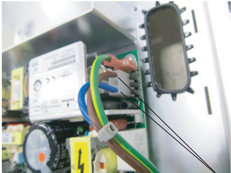
Verify AC potential between these two points
