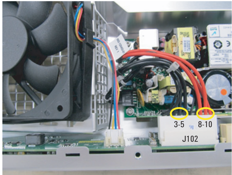
Figure 13 Verify power supply DC output
