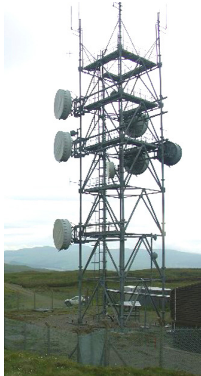
Figure 6a. Microwave repeater showing multiple co-located antennas. 3
