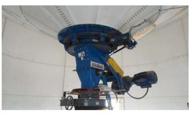
Picture 2: Reclaimer screw system installed at the bottom of the silo
