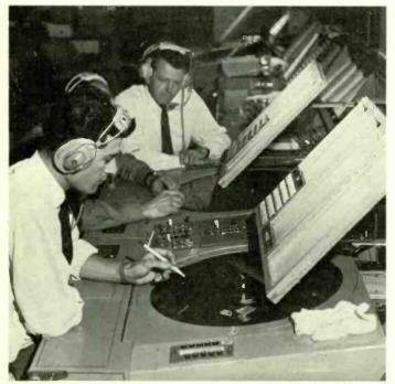
Controllers at work during a Mediator simulation. Recently the equipment was used to determine which was the best site for London's third airport from an air traffic control point-of-view; Foulness came out tops.
