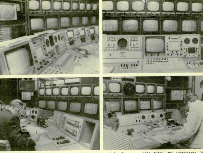
The master control desk at Thames Television's new centre in Euston is boomerang-shaped and has positions for the lines engineer (top left), the engineer in charge who performs a quality control function (top right), and the network switcher (bottom left). The monitor bank facing the desk has a row of 14-in. monochrome monitors and a row of colour monitors underneath. These preview incoming sources, check the passage of signals
